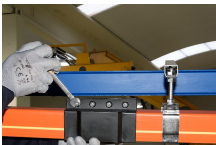
Fit and tighten the screws of the joint EMPC-4 splices. Check correct alignment between beam and power line.
