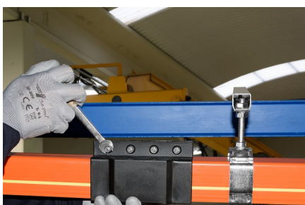
Fit and tighten the screws of the joint EMPC-4 splices. Check correct alignment between beam and power line.
